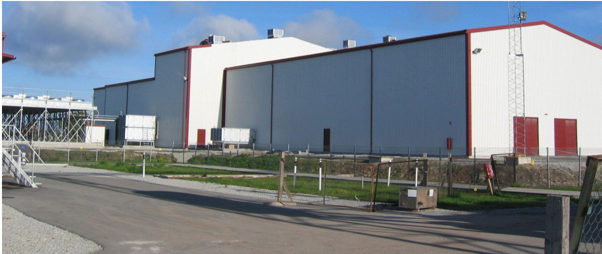
The Harku high-voltage direct current converter station, the Estonian side of EstLink 1
